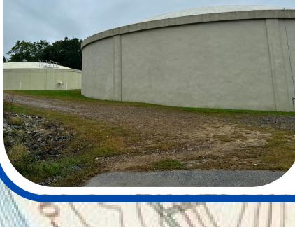
Water storage tanks play a crucial role in the distribution of water from a treatment plant by providing a reserve supply, ensuring consistent water pressure, and serving as a buffer during peak demand periods. Our treatment plant has a 1.3 and 2.0 million gallon tank on site at our plant.
