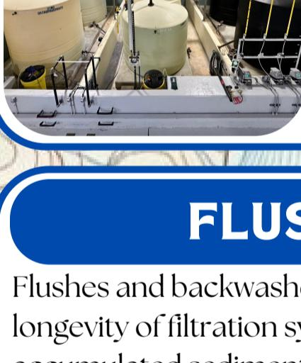
An important step in water treatment is the use of chemicals for various purposes. The chemicals we use are: Sodium Hypochlorite for disinfection, Caustic Soda for pH adjustment, Zinc Orthophosphate for corrosion control, Alum for coagulation, and Sodium Fluoride for oral treatment.
