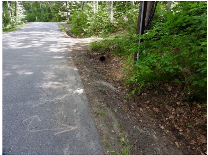
Example of a road ditch with accumulated sediment and vegetation scraped out to maintain hydraulic capacity, as part of the town's maintenance practices.
