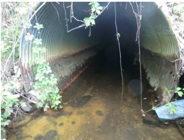
Typical undersized culvert
