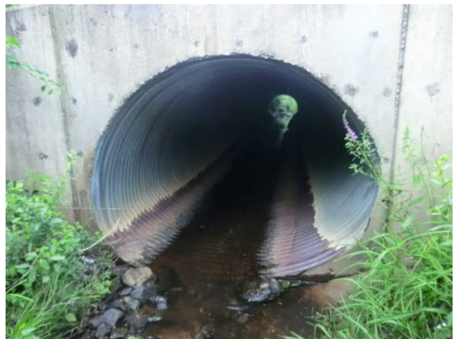
Another typical undersized culvert:
