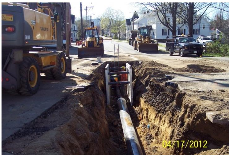
New water main inside a steel sleeve that was placed under the railroad tracks
