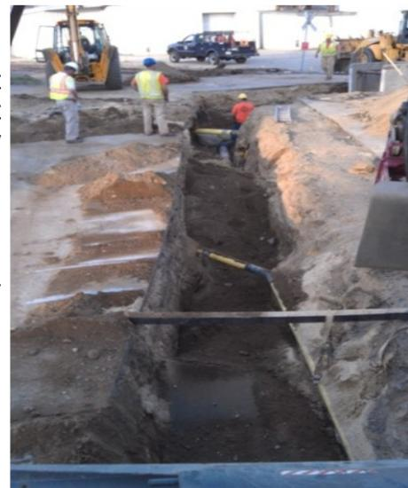
New water main had to be placed under the existing gas lines
