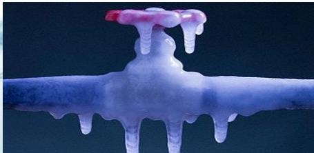
If the temperature inside a house gets below 32 degrees Fahrenheit (0 degree Celsius) it's likely that the water supply pipes and the drain traps will freeze. When water freezes it expands 9 percent, and if there is no room for expansion it's possible that the pipe will develop a crack and eventually leak once the ice thaws out. Fixing a burst pipe can be expensive, but the damage from uncontrolled water leakage can easily reach into the thousands of dollars.
