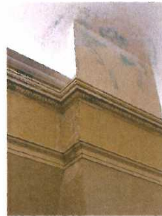
South chimney water penetration in the Periodicals Room, Main Level.
