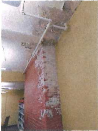
South chimney water penetration in the Children's Room, Lower Level.
