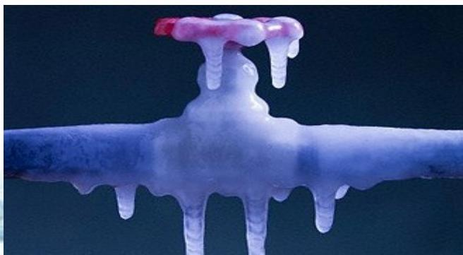
If the temperature inside a house gets below 32 degree Fahrenheit (0 degree Celsius) it's likely that the water supply pipes and the drain traps will freeze. When water freezes it expands 9 percent, and if there is no room for expansion it's possible that the pipe will develop a crack and eventually leak once the ice thaws out. Fixing a burst pipe can be expensive, but the damage from uncontrolled water leakage can easily reach into the thousands of dollars.
