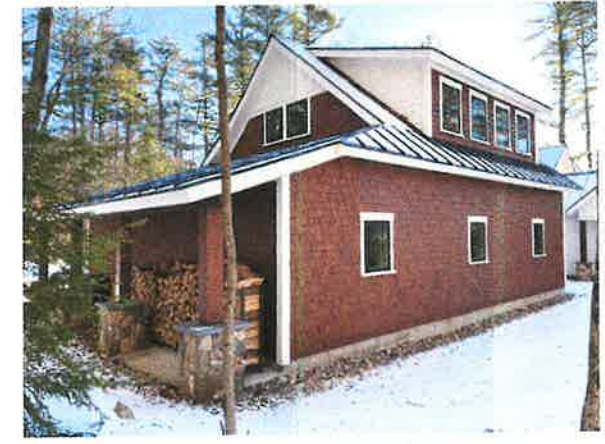
REAR VIEW LOOKING SOUTHERLY
