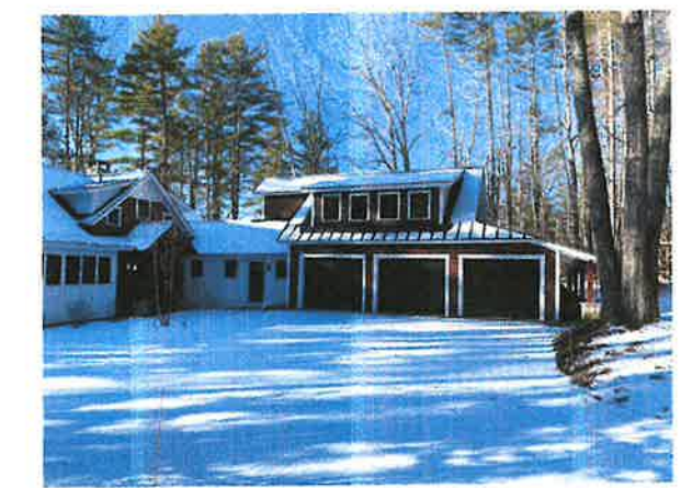
FRONT VIEW LOOKING WESTERLY
