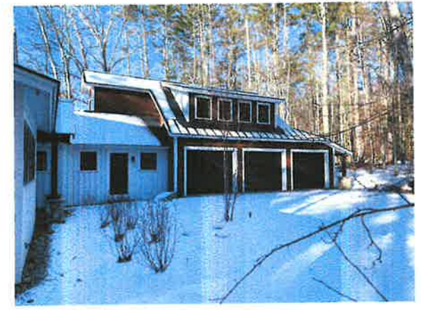
FRONT VIEW LOOKING WESTERLY
