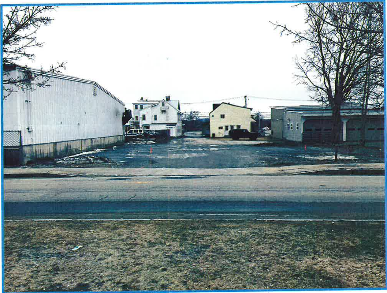
View looking northwest at 60 Mechanic Street.
