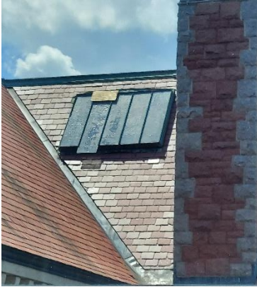
1. Skylight with plywood covering.
