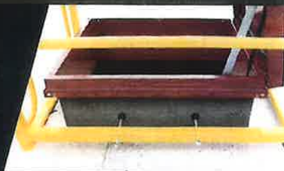
SIMPLE COMPRESSION FIT ON CURB
